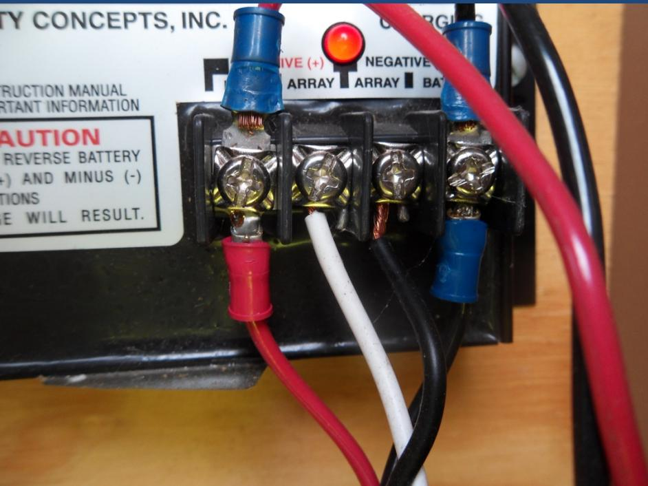
Multiple wires in a terminal connector
