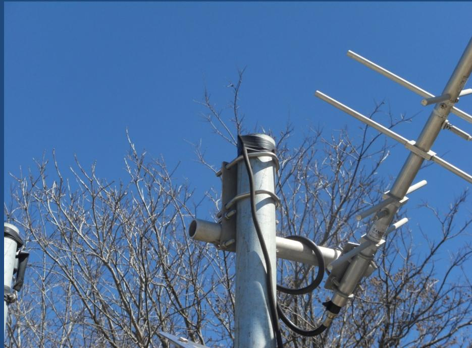
**Careful with metal straps as they could cut into the outer cable jacket**
